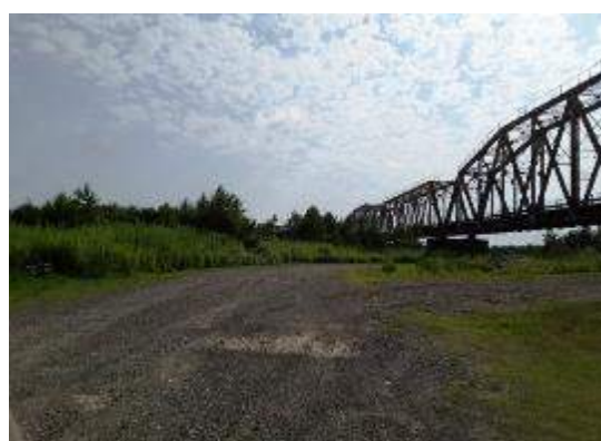
Vegetation near railroad bridge
