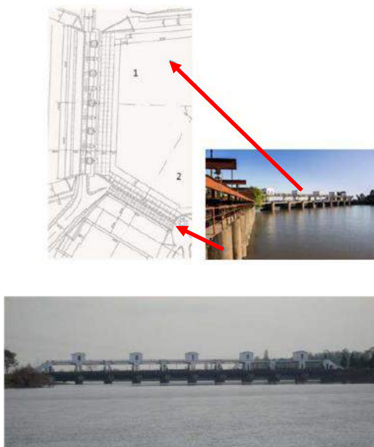
Figure 63. Diversion Dam on the Rioni River
