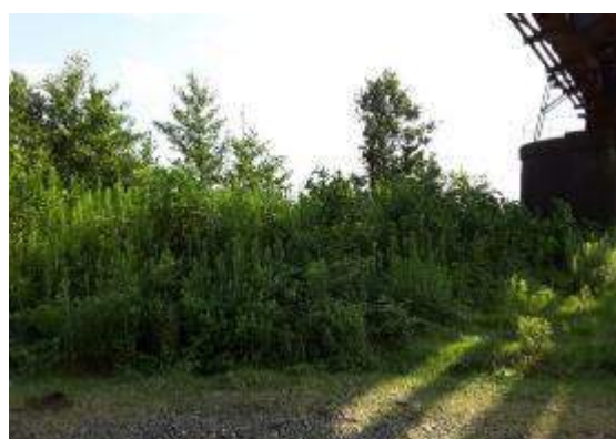
Vegetation under railroad bridge
