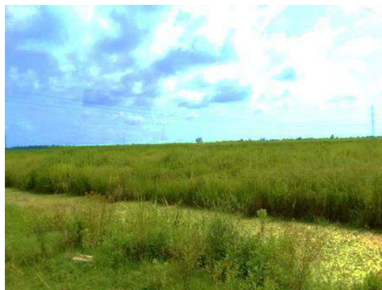
Drainage canal overgrown with amorpha
